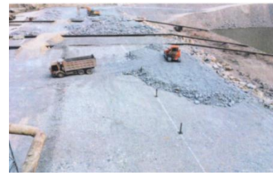
(a) Spreading the rockfill
