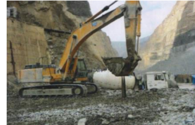
(b) Sprinkling the composite grout
