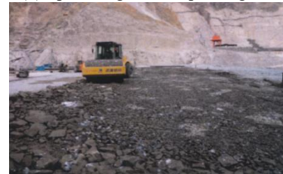
(c) Rolling compaction
